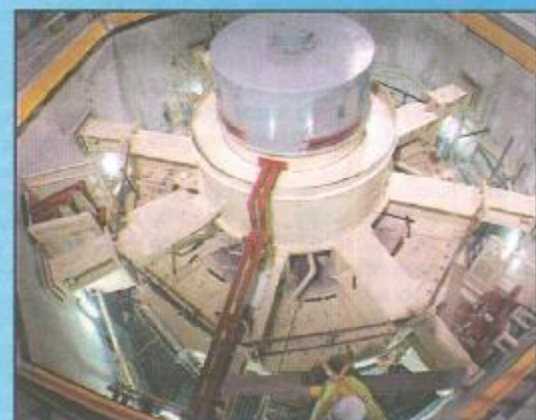
Above: The tops of the 2 Generators which show the Exciters on the Turbine Floor.
