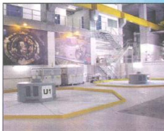
Above: The tops of the 2 Generators which show the Exciters on the Turbine Floor.
